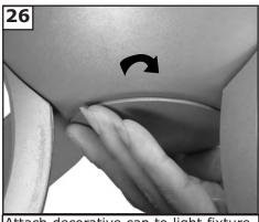
Attach decorative cap to light fixture by twisting into place.
